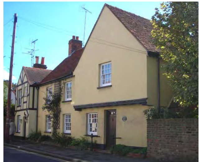
Fig. 42 Anchor Cottage, 17 High Street.
