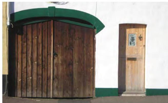
Fig. 25 Carriage arch, Prospect Cottages.
