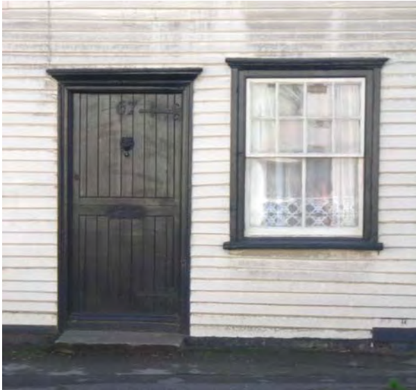
Fig. 20 Weatherboard and simple architraves, No. 67 High Street.
