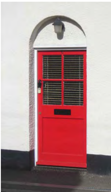
Fig. 21 Recessed doorway, no. 6 High Street, within a Victorian brick arch.
