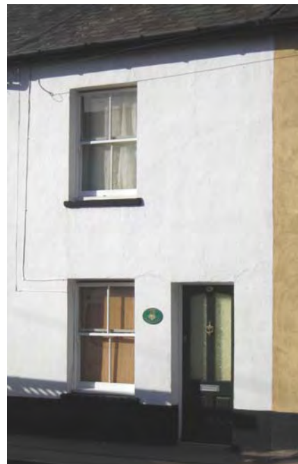
Fig. 22 Simple Victorian terrace façade, no. 76 High Street.
