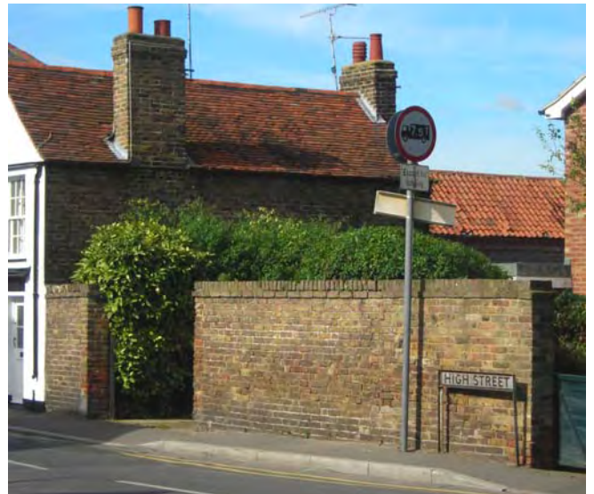
Fig. 23 Stock brick boundary wall, 2a High Street.
