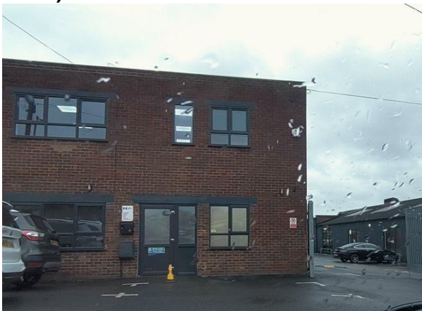
Figure C19: Brook Road Industrial Estate (ELS04).
