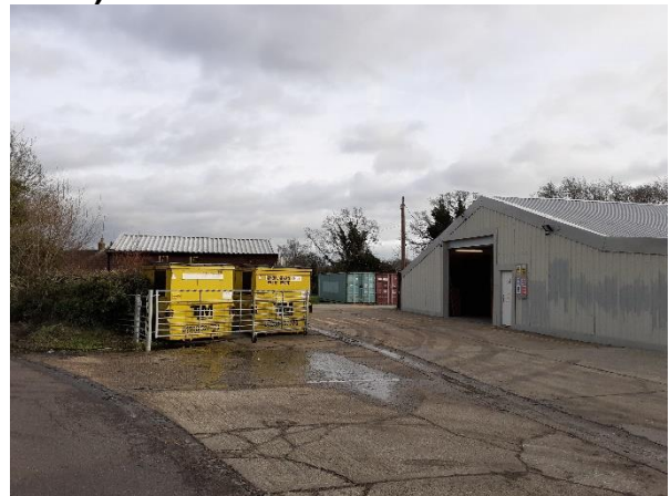
Source: Rochford District Council (2024)
