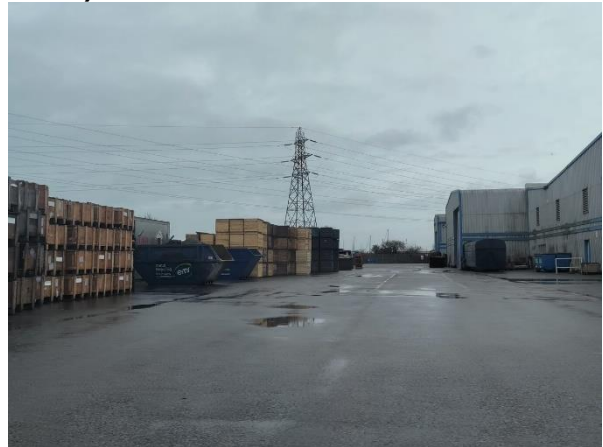
Figure 35: Purdey's Industrial Estate (ELS10).
