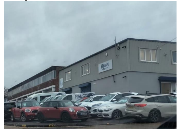
Figure C20: Brook Road Industrial Estate (ELS04).
