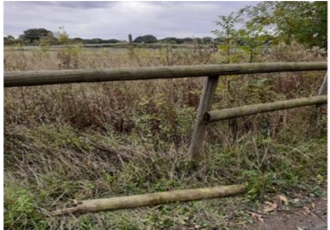
Figure 47: some areas need maintenance
