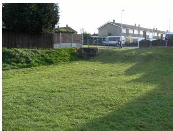
Figure 10-4: Albany Road, Flood Storage Area, Wickford
