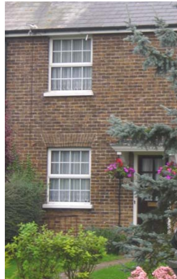
Fig. 45 Replacement UPVC windows, no. 17 Churchend.
