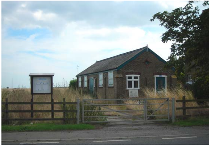
Fig. 36 QinetiQ estate office.
