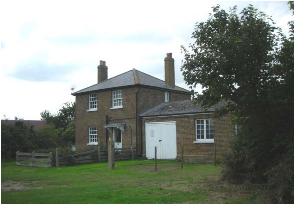
Fig. 32 No. 19 Churchend, former blacksmith's cottage and workshop.
