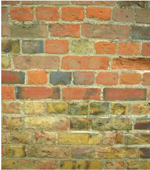
Fig. 18 Local soft red and yellow stock brick, laid predominantly in English bond, on old farm building.
