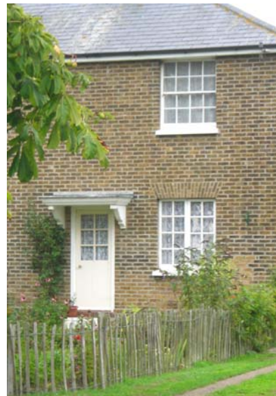
Fig. 19 Small paned casements and sash windows, traditional door with simple canopy, no.18 Churchend.
