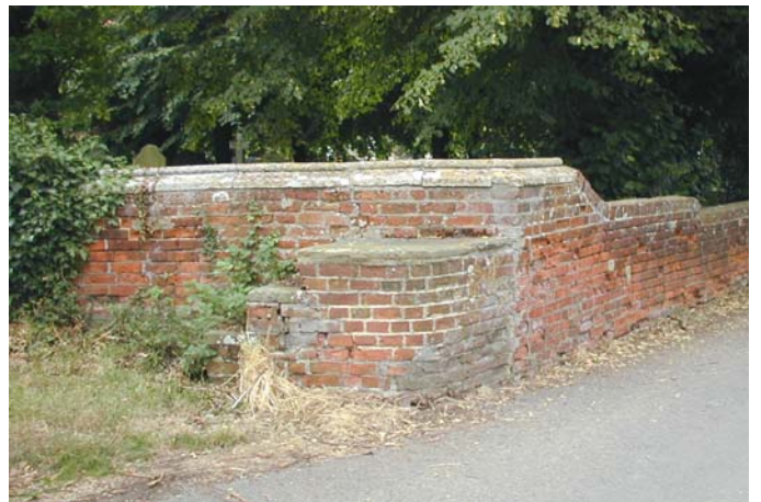
Fig. 28 Mounting block on south west corner of churchyard wall.
