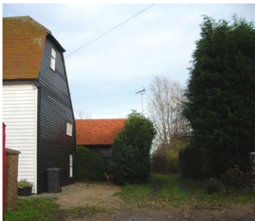
Fig. 31 Rear access, the Old Post Office.
