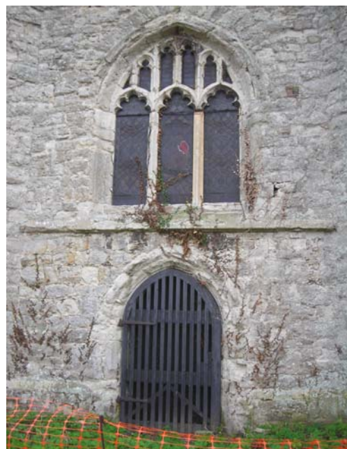
Fig. 32 West window and door, currently barriered-off.
