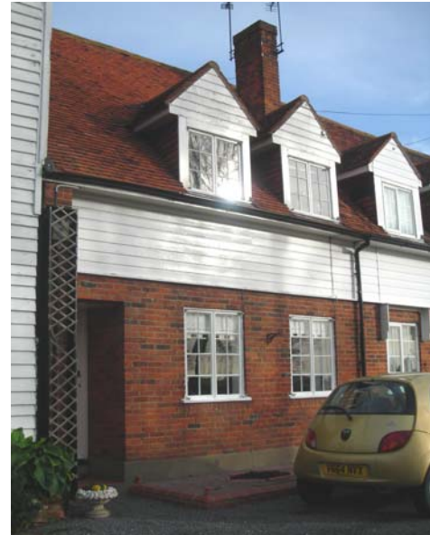
Fig. 20 No. 1 Punchbowl Cottages, with metal windows and timber weatherboard.
