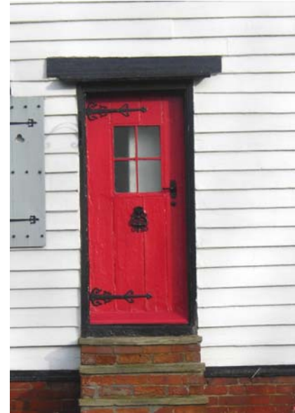
Fig. 14 Painted boarded door, Post Office Cottages.
