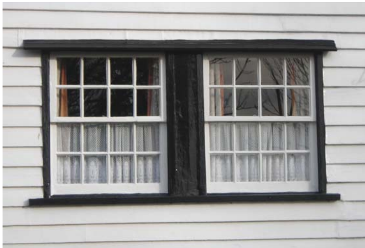
Fig. 15 Small paned sash windows with pentice,
