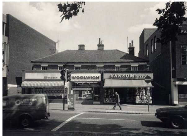
Fig. 10 High street, nos 57-61, before redevelopment.
