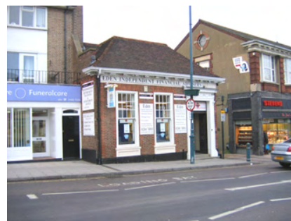
Fig. 40 High Street, no. 102, former Westminster Bank building.
