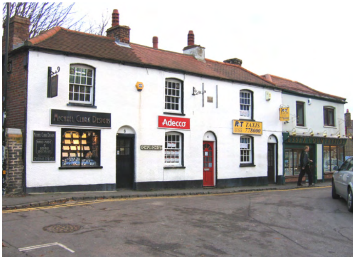
Fig. 20 Nos 4-8 Church Street.
