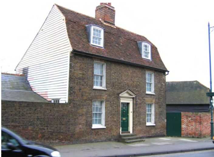
Fig. 13 No. 18 Hockley Road, an 18th-century house provided with a stock brick façade in the 19th century.
