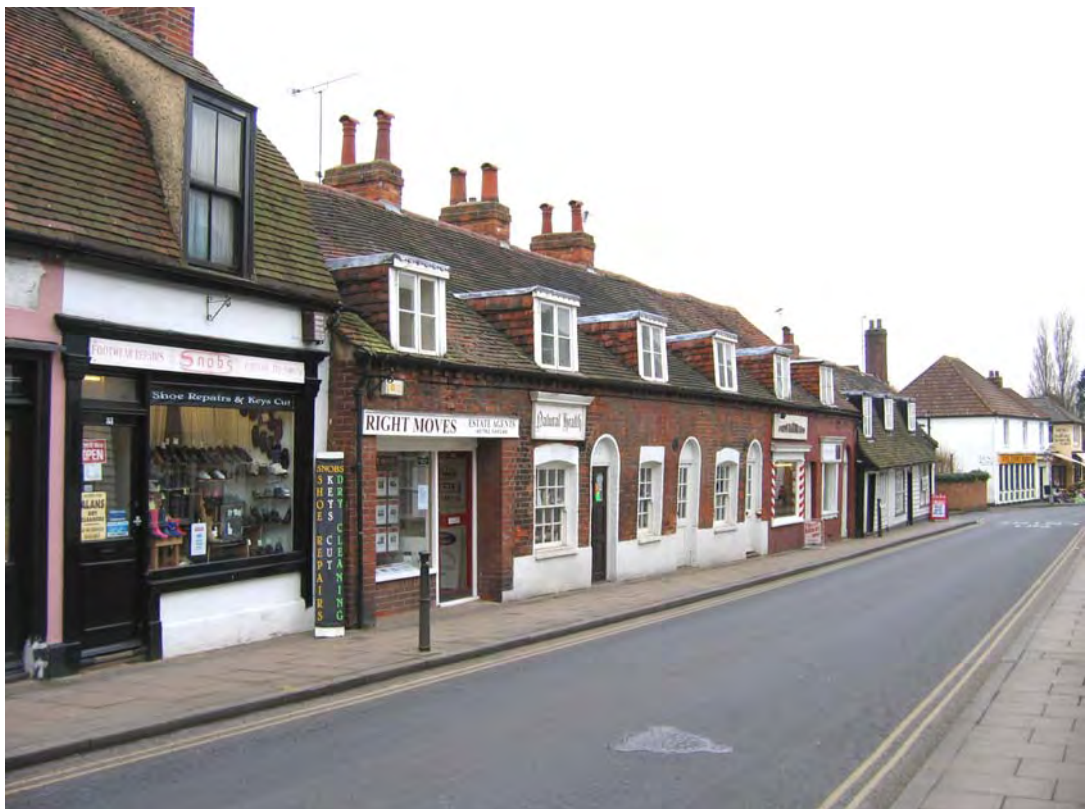
Fig. 45 West Street, cottages at west end (nos 53-69).
