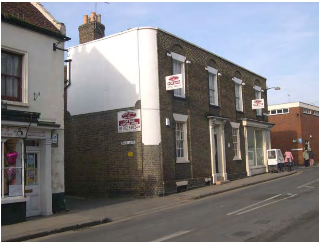
Fig. 25 No. 1 South Street.
