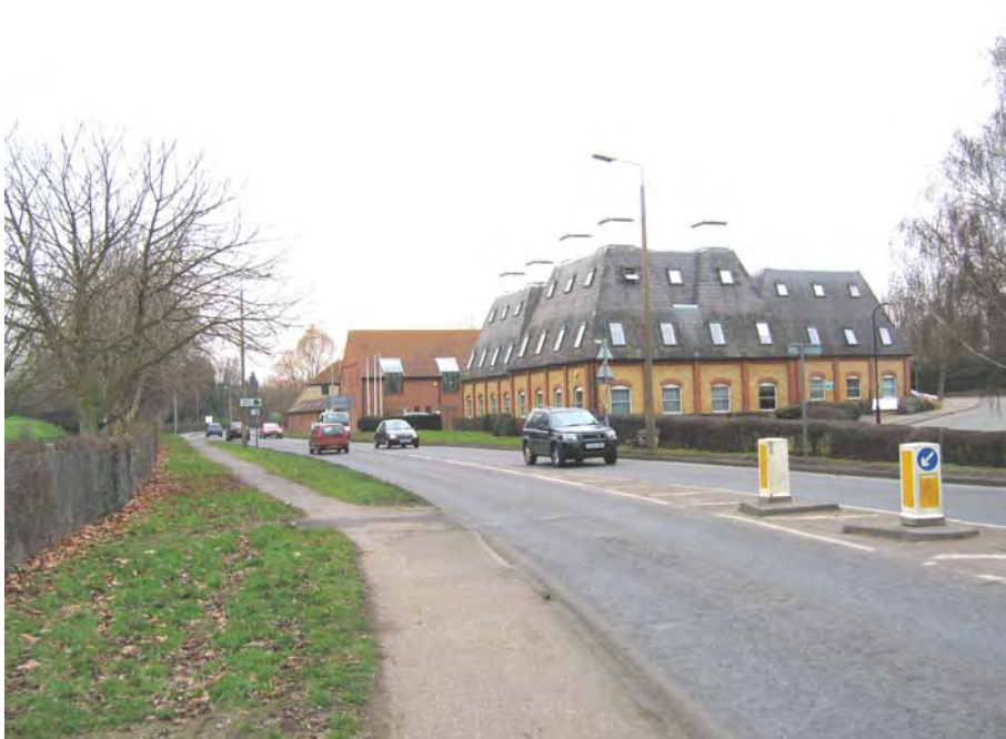
Fig. 30 Bradley Way and Canewdon House.
