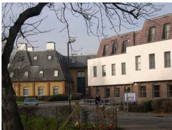
Fig. 31 Locks Hill, Cottis House and Canewdon House.
