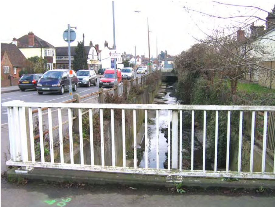
Fig. 36 West end of West Street, the concrete lined conduit for the Iron Well Stream.
