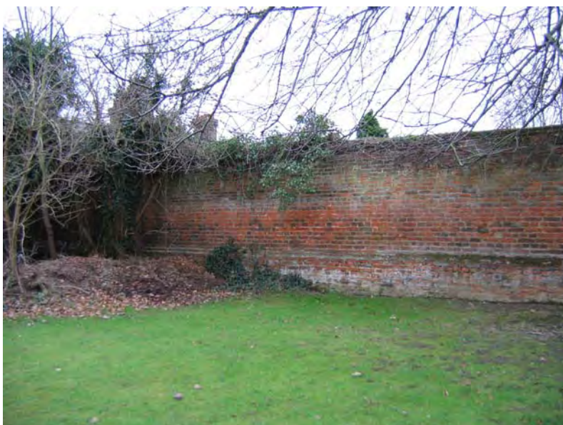
Fig. 18 Hall Road, one of the least overgrown parts of the Tudor boundary wall.
