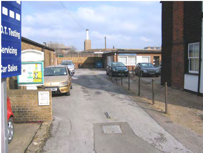
Fig. 35 West Street, depressing view between Whittingham's garage and Sovereign House to the parish council offices. In the background, the former hospital boiler house.
