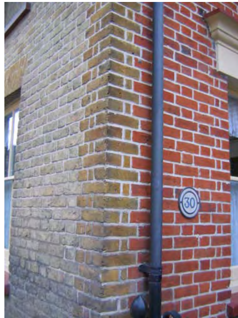
Fig. 11 Angle of nos 30-32 South Street. White bricks were used for the façade, with stocks for quoins and window lintels, and red bricks in the side.
