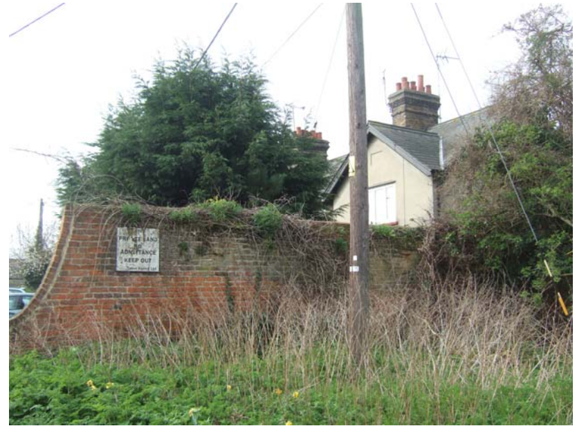
Viewpoint 10 (Looking south/south west)
